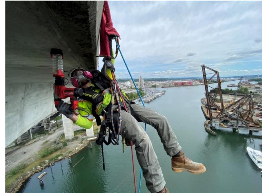
SPRAT Ropes Access to obtain exterior concrete samples
